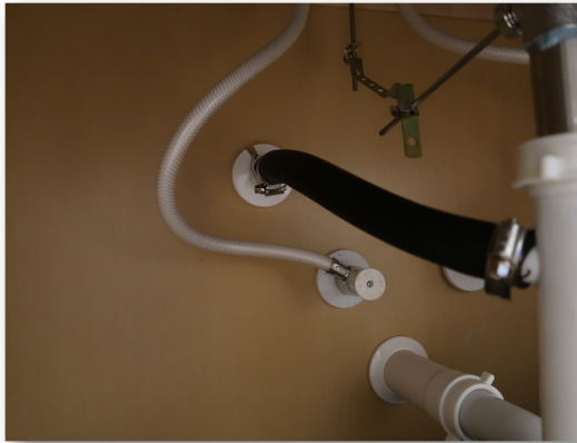
Primary Drain Line
