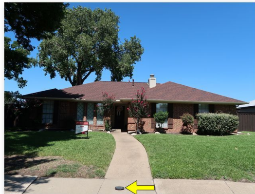
38. The city sewer line cover is protruding above the walkway floor.
