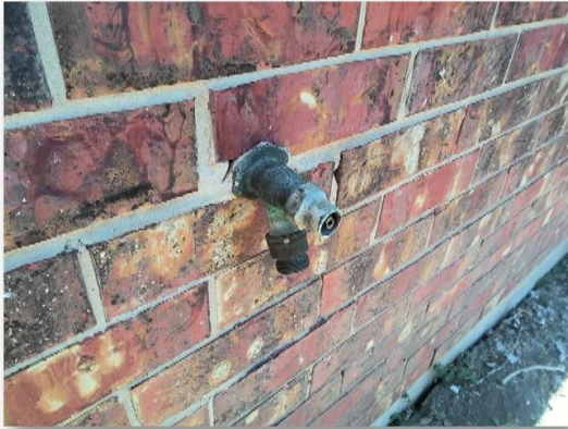
54. One of exterior faucet missing the handle.
