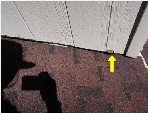
34. There is paint chipping on the chimney sidewall, and paint is peeling around the rain cover.
