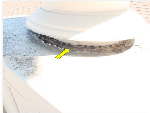
34. There is paint chipping on the chimney sidewall, and paint is peeling around the rain cover.
