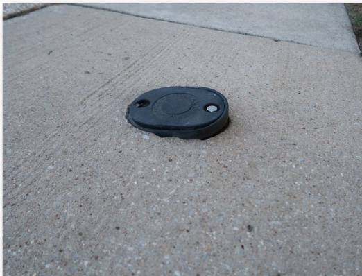
38. The city sewer line cover is protruding above the walkway floor.
