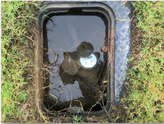
Water Meter Location : in underground box near the sidewalk Water Shut Off Location : in Garage wall
