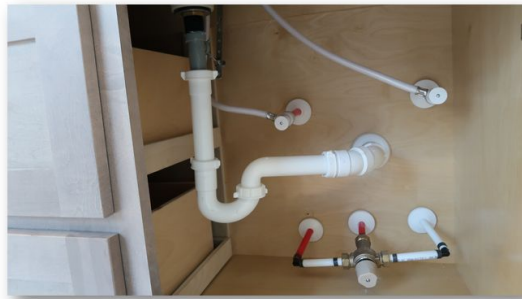
Wash machine drain line Min 18" to Max 30" or 42" from bottom.
