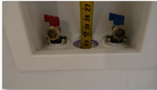
Wash machine drain line Min 18" to Max 30" or 42" from bottom.
